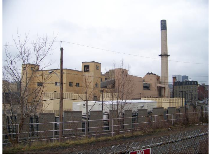
View from the northwest
