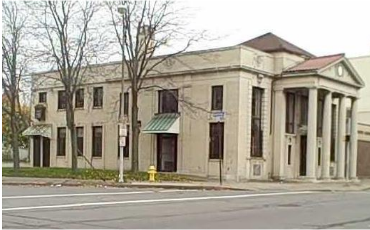
175 Lyell Avenue, former bank building
