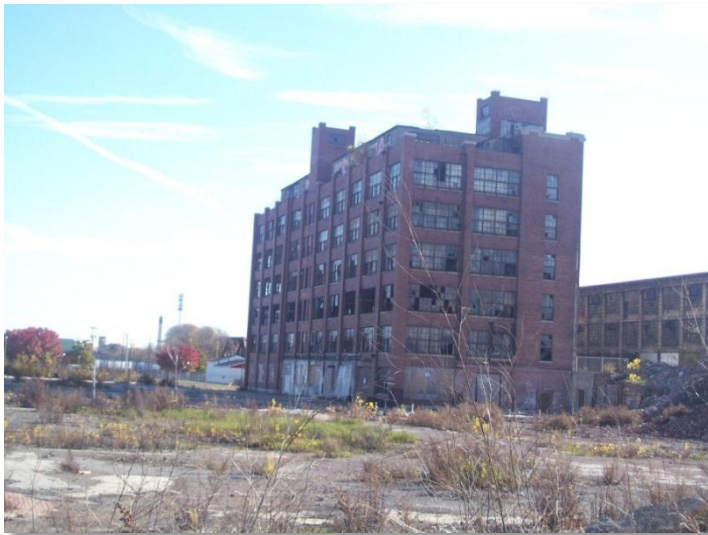
Dilapidated buildings on the Orchard-Whitney Site
