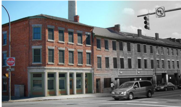
Rehabilitation of the Teoronto-Smith Block Historic District
