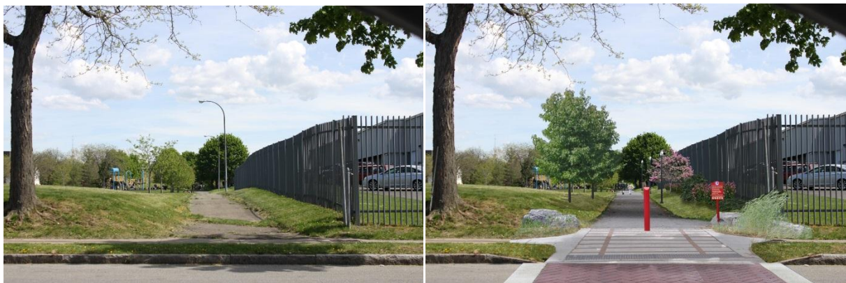
Existing Trail at School #5 Looking South, Before and After Improvements
