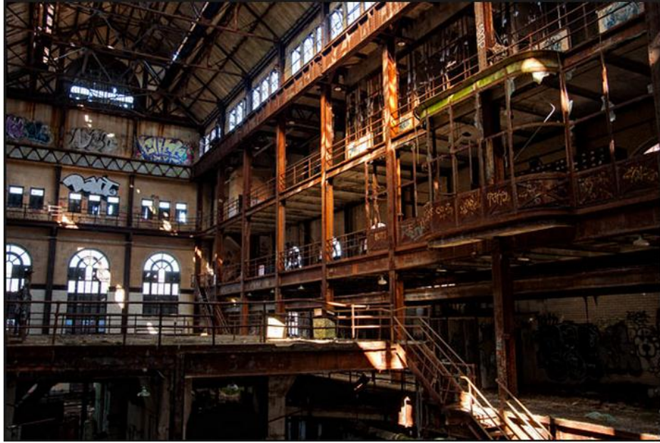
Glenwood Power Plant, Yonkers
