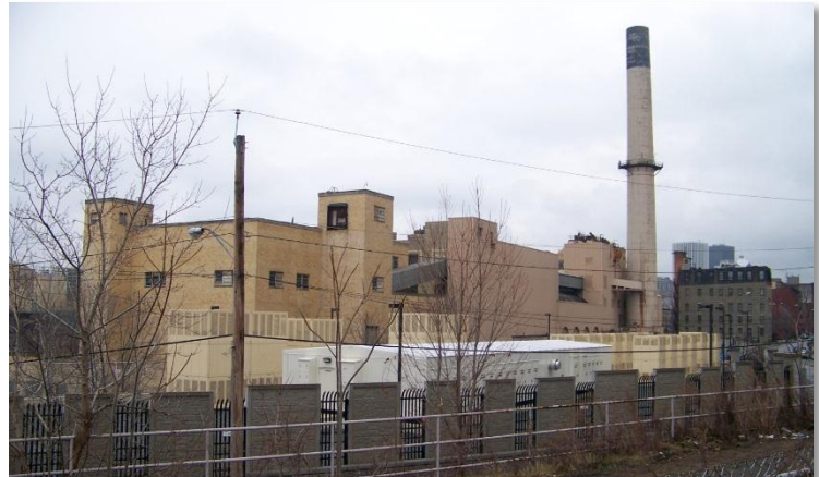
Rochester Gas & Electric's BeeBee Station from Mill Street
