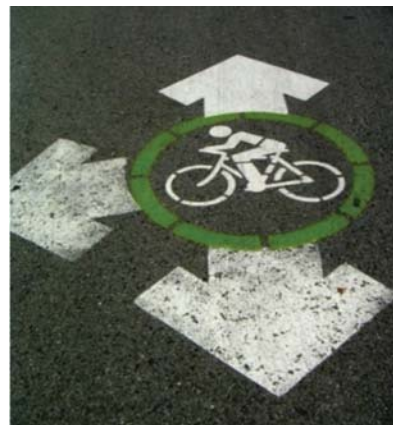
Bicycle boulevard pavement markings are an opportunity to develop unique branding with wayfinding
