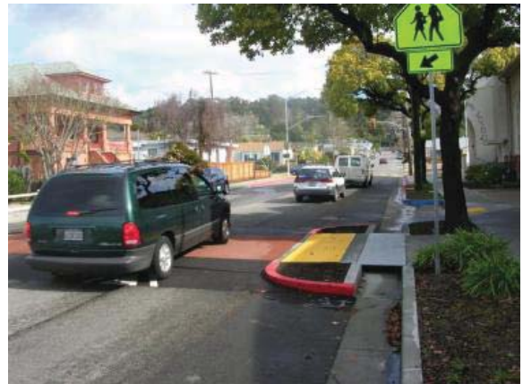
This raised crosswalk incorporates curb extensions that facilitate drainage. Source: East Bay Bicycle Coalition
