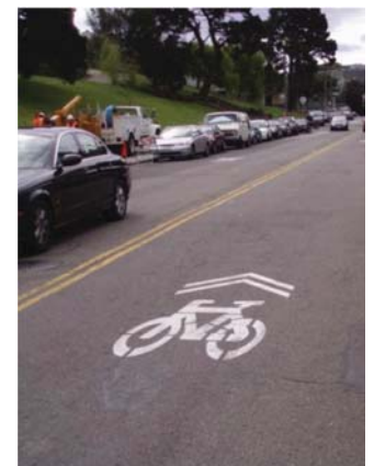
Shared Lane Markings encourage motorists to share the road
