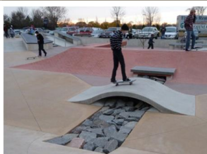
Recycled Granite Drainage Swale
